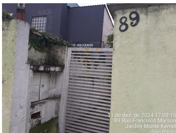
Foto 17 – Rua Francisco Marson, 89.
